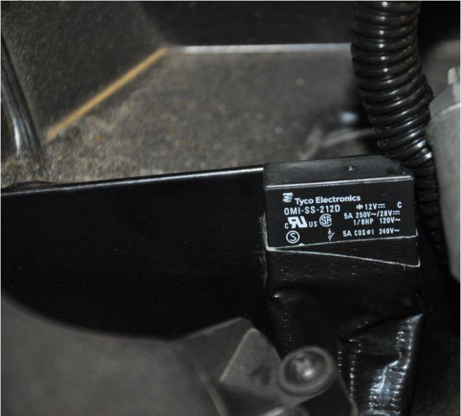
Tap in fuse box
