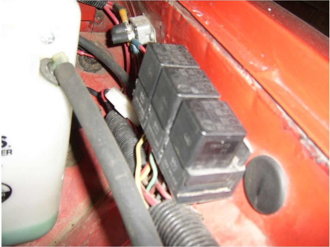
Relays for fans and a/c compressor
