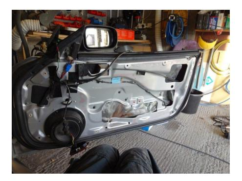
Then wound the glass to this position and removed the earth from the battery.
