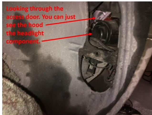
Proof that only the access door was removed
